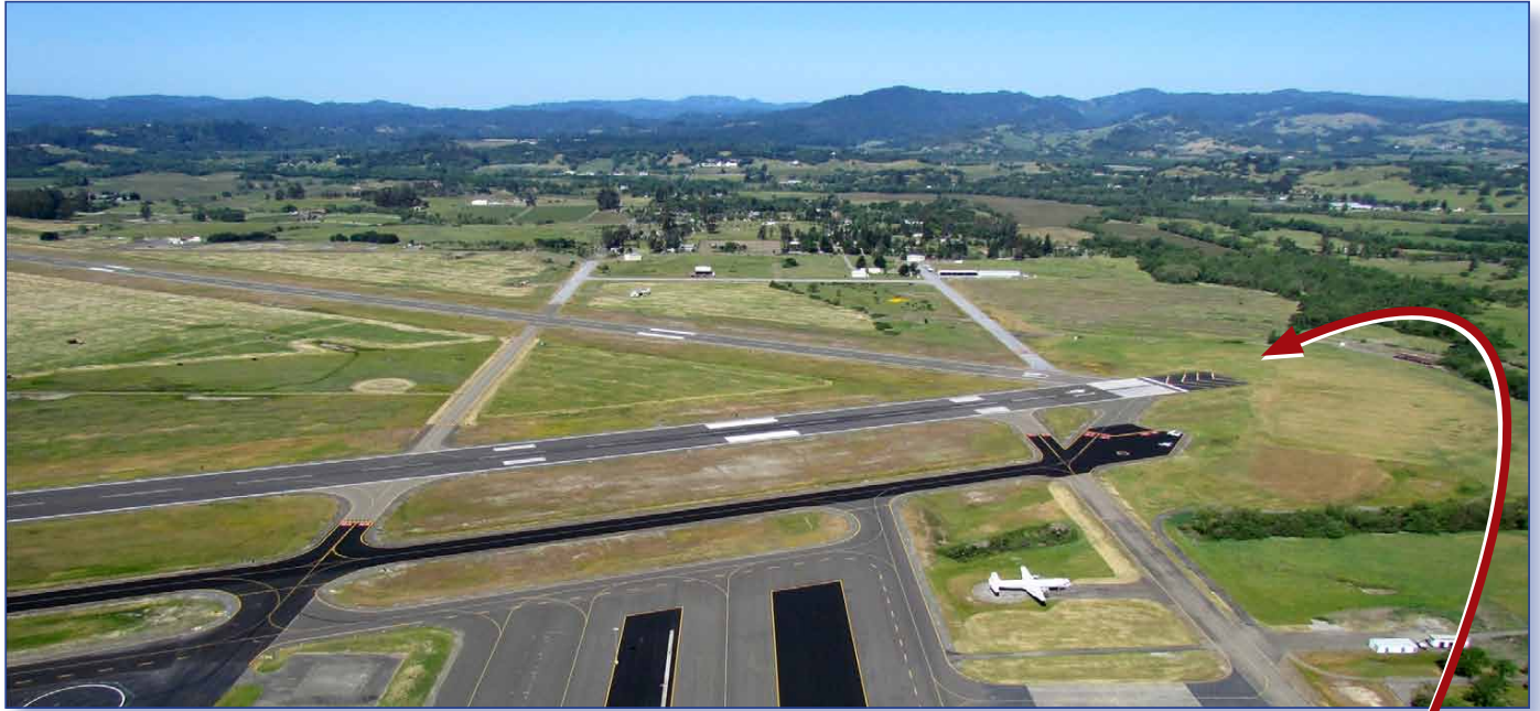
STS runways seen from the air looking west. The coupled runways will be improved to meet current safety standards.
